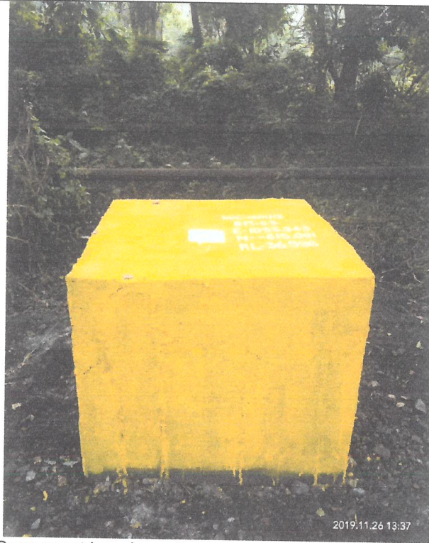
Permanent bench mark constructed at complex area
