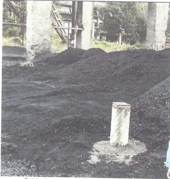
Grid pillar established near Coal heap
