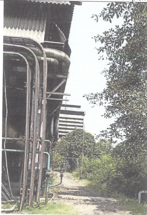
Cooling tower at complex area
