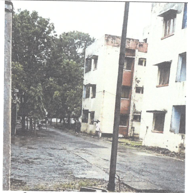
Control building inside the complex area
